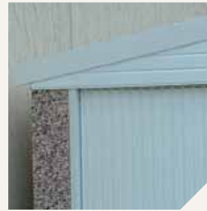
White PVCu fascias and vergeboards
