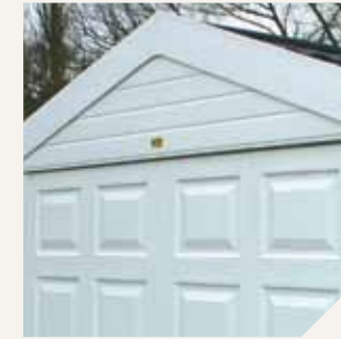
White PVCu fascias and vergeboards
